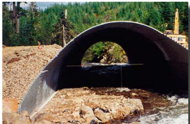
Figure 7.5—Multiplate open-bottom pipe arch.
