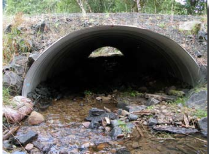
Figure 7.3—1-piece corrugated metal pipe arch (embedded).
