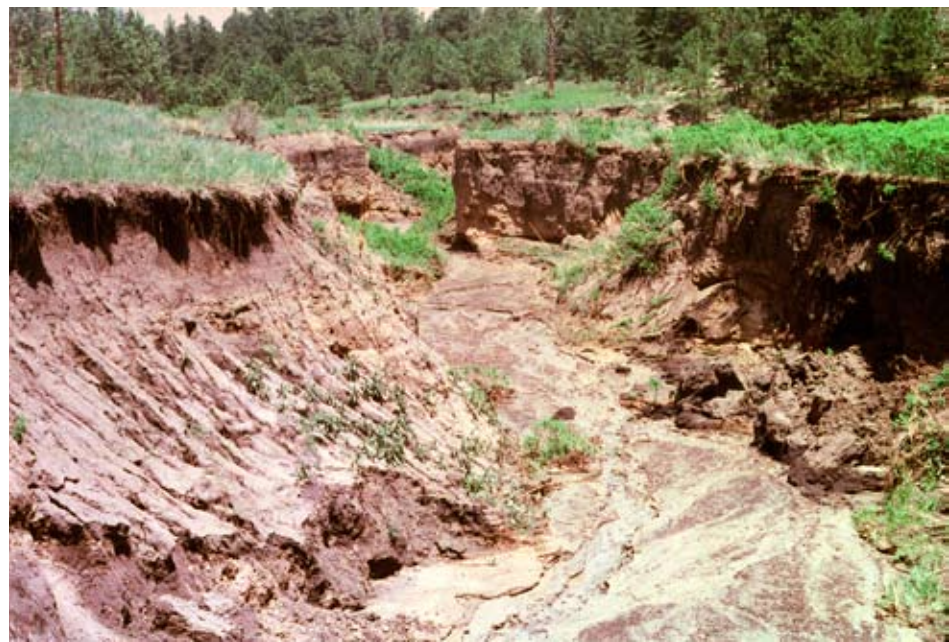
Figure 4.6—Channel widening after recent incision, eastern Colorado.
