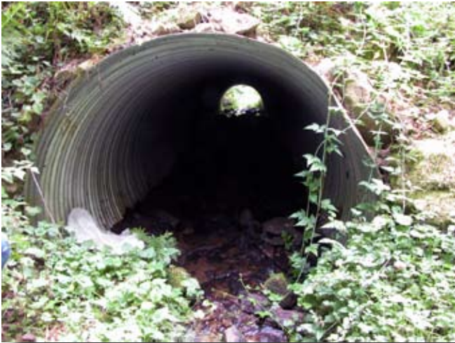
Figure 7.2—1-piece corrugated metal pipe (embedded).
