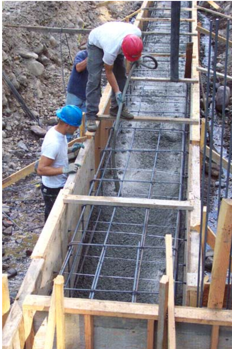
Figure 8.10—Concrete forms and reinforcing during concrete pour.
