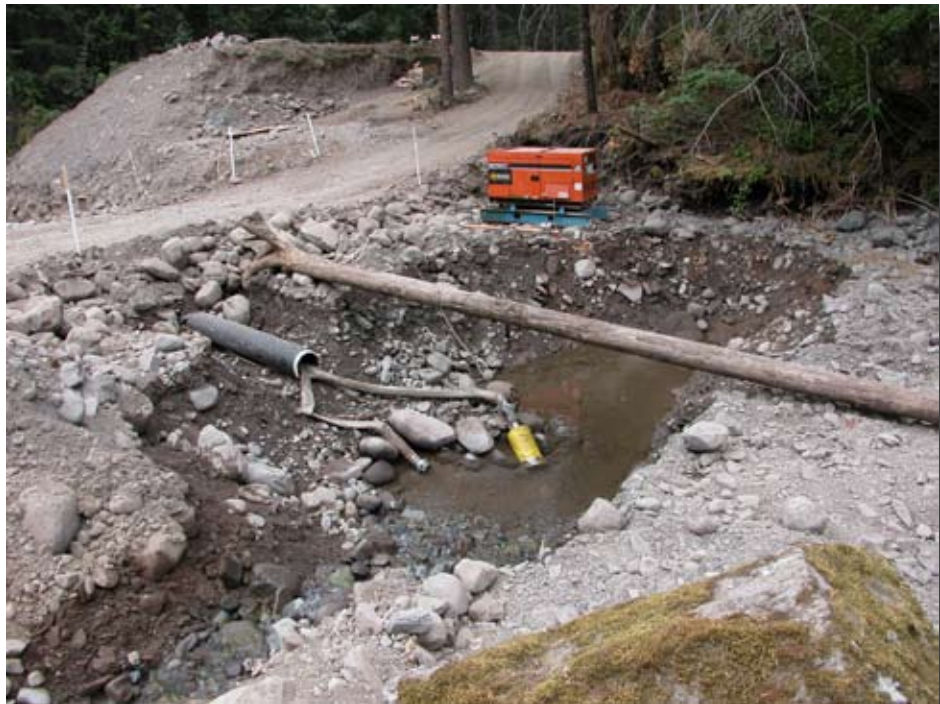
Figure 8.5—Upper sump collects water that bypasses or seeps through the diversion dam.
