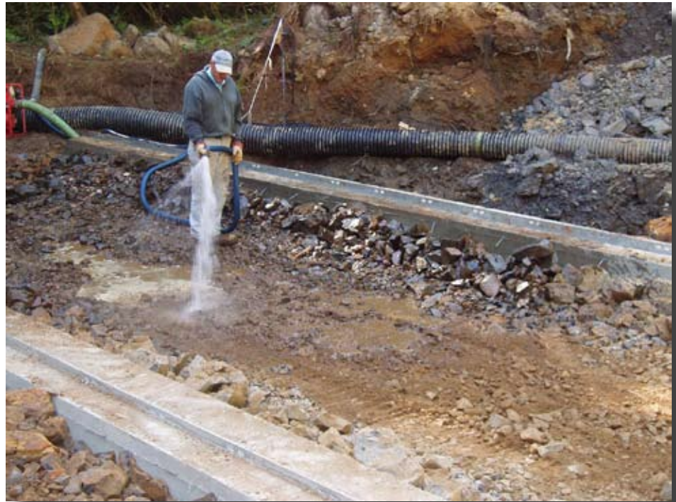
Figure 7.14—Washing filler material into the voids in the stream-simulation bed.
