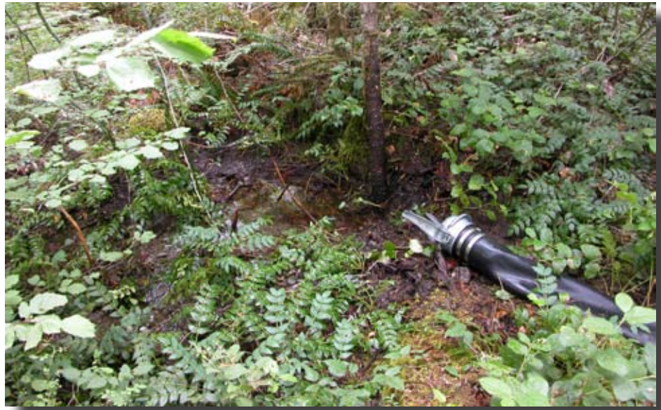
Figure 8.8—Natural filtration on the forest floor isolated from the stream channel is one means of treating sediment-laden water.
