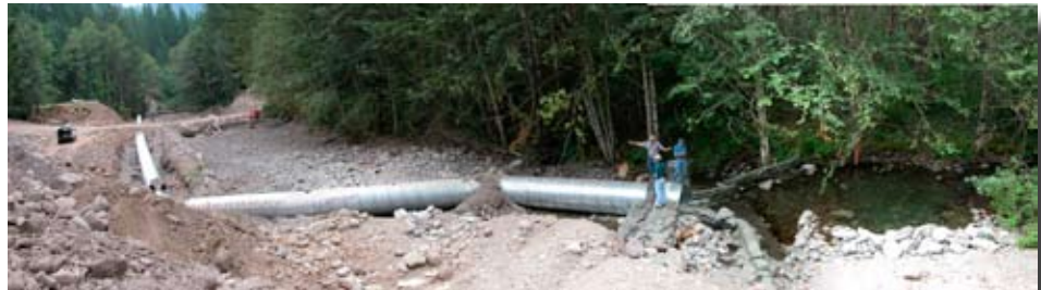
Figure 8.4. Diversion dam and gravity pipe bypass system. Bypass road is visible in the background, and excavation in main road is just beyond it.
