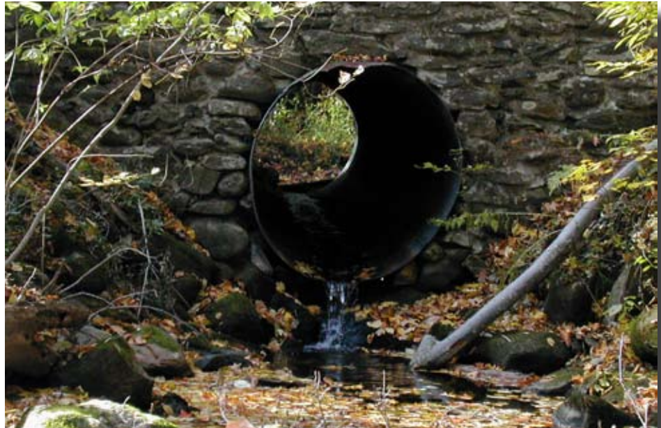
Figure 1.15—Many crossing structures are narrower than the stream and block fluvial processes that maintain aquatic habitats. The structures also impede aquatic species passage. Photo: Scott Jackson, University of Massachusetts.
