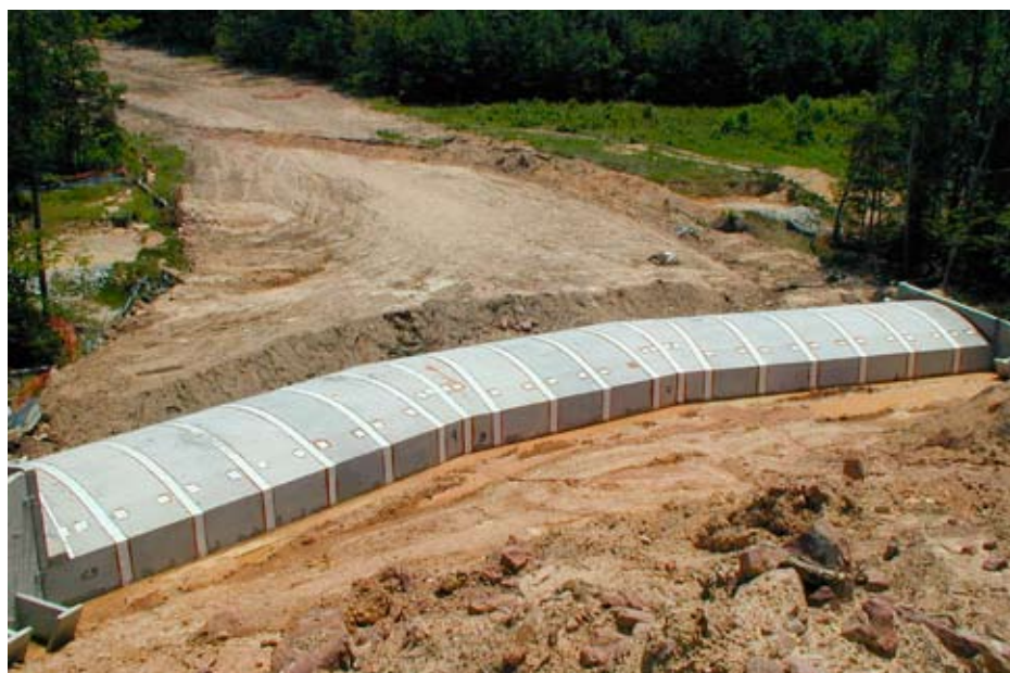
Figure 6.5—Curved concrete pipe installation at Arrington Development, Durham, North Carolina, June 2001. (Pipe is 142 feet long, with a 24-foot span and a 7-foot rise.) Courtesy of CON/SPAN Bridge Systems.
