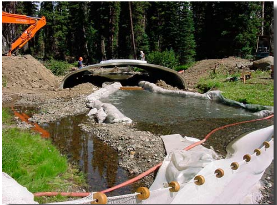
Figure G.11—South Fork Desolation Creek construction site showing block nets.
