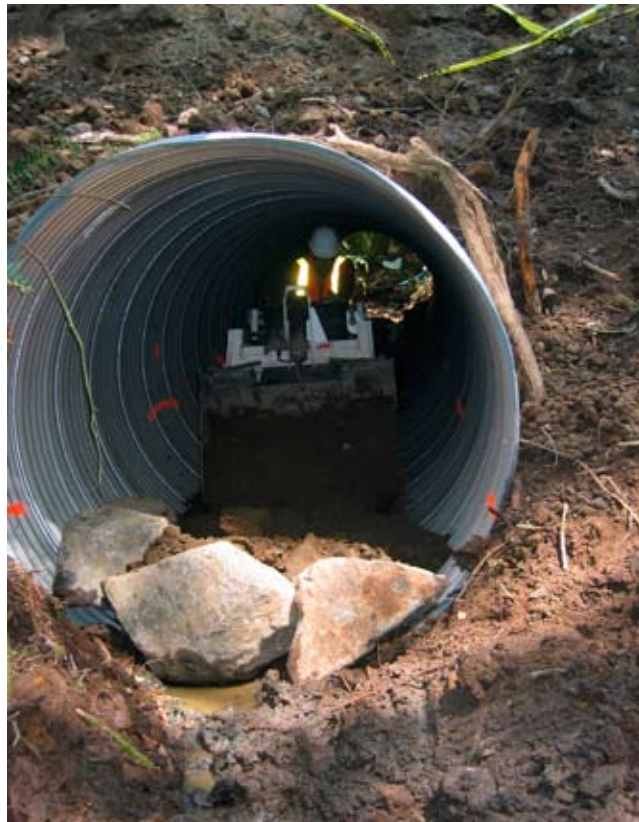
Figure 7.13—Hand labor walk-behind equipment.
