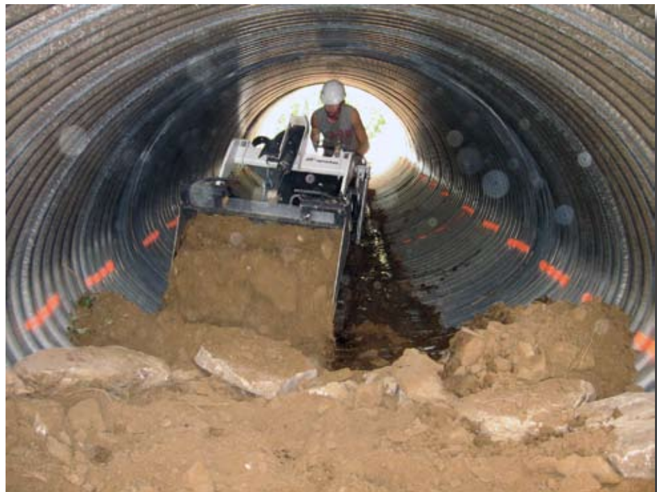
Figure 8.15—Bobcat placing bed material to marked elevation.
