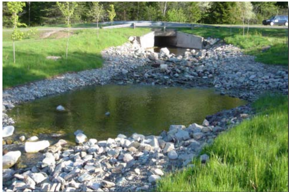
Figure F.3—Rock riffle used to backwater the outlet of a box culvert on Dickson Brook, Bay of Fundy, New Brunswick, Canada. Photo courtesy of Dr. Robert Newbury, Newbury Hydraulics, Okanagan Centre, British Columbia, Canada.
