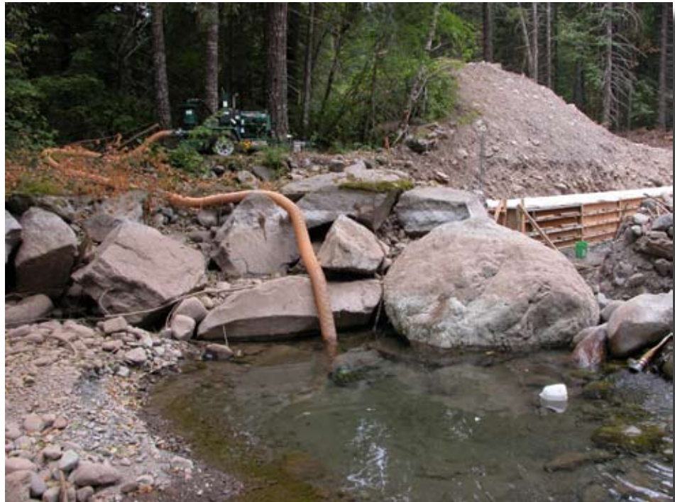
Figure 8.6—Lower sump collects water bypassing the construction. The hose on the right is discharge from the upper sump. The water is pumped from the sump to a treatment area where the water is dispersed in the vegetation.
