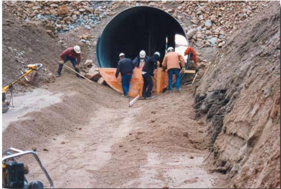
Figure 7.9—Shaping culvert bedding.
