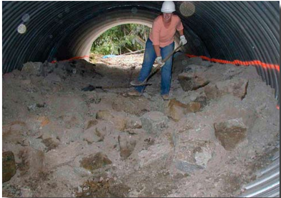
Figure 8.16—Assuring proper cross-section shape, rock-band spacing and placement of channel rocks and footers often require hand work.
