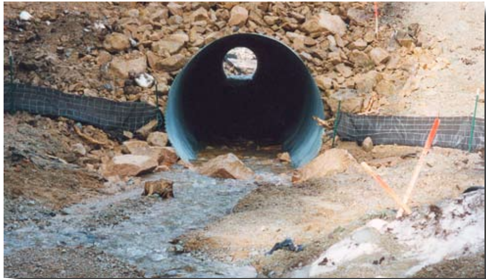
Figure 7.22—Typical silt-fence installation.
