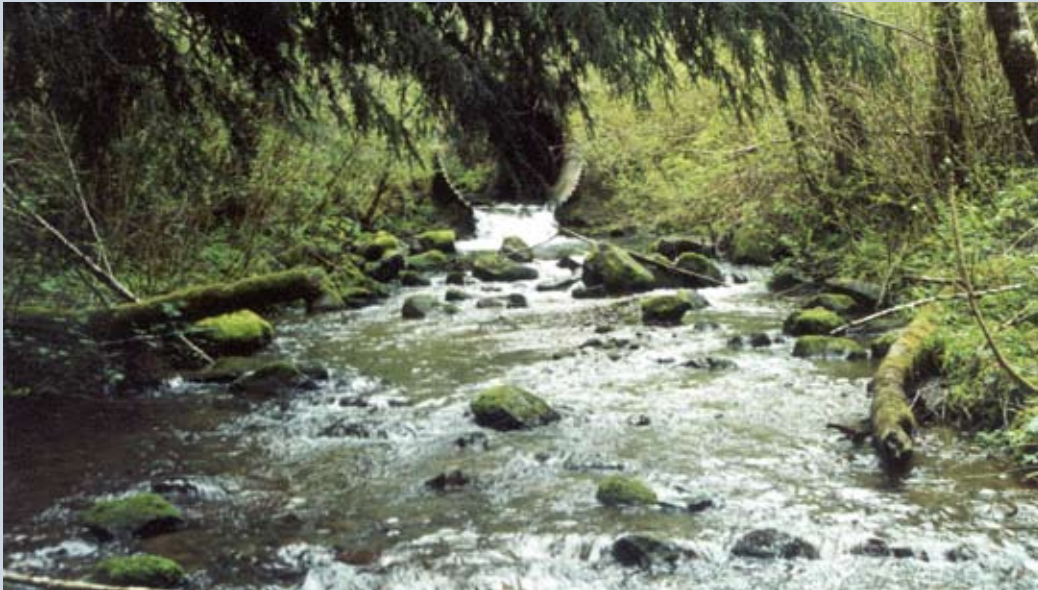
Figure 5.11—Outlet of existing culvert on Newbury Creek, Olympic National Forest, Washington.
