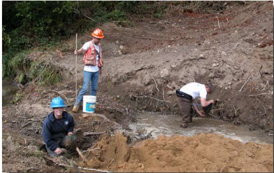
Figure G.13—Capturing aquatic organisms by hand as the site is dewatered.
