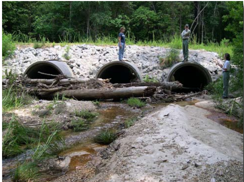
Figure 3.3—Multidisciplinary project team on initial reconnaissance of a project site.
