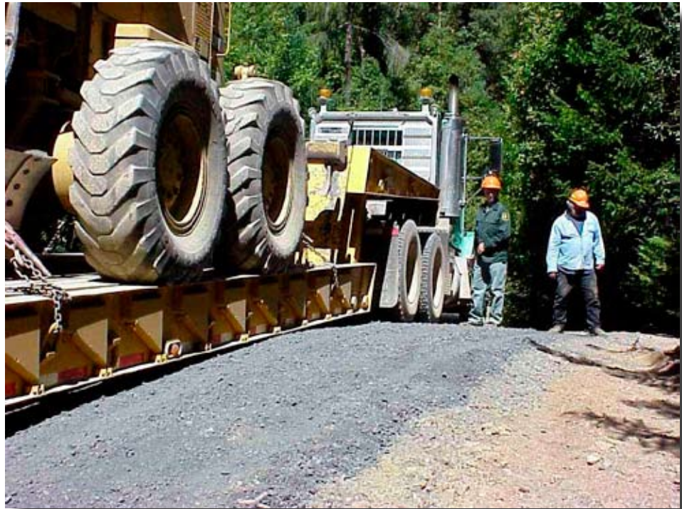
Figure 8.19—The grade change at this dip is too severe to accommodate a lowboy, which has high-centered on top of the dip.
