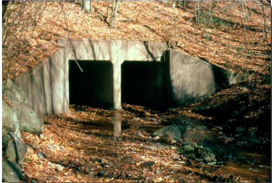
Figure 1.23—Lack of a low-flow channel results in insufficient water depth in these box culverts. Photo: Scott Jackson, University of Massachusetts.
