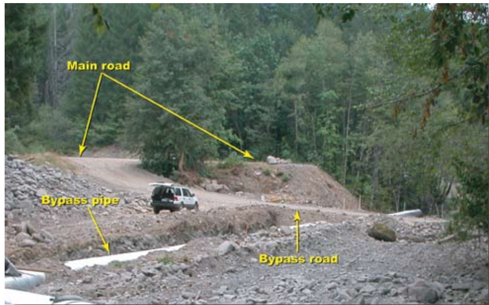
Figure 7.12—Typical construction site traffic bypass.
